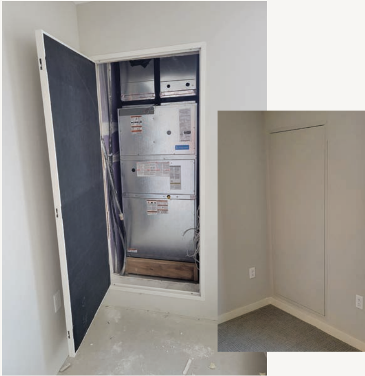
HVAC Access Door installation
